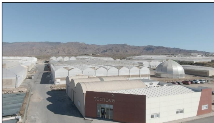
Figure 1. General view of the Experimental Centre.
